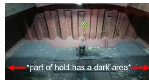
Insufficient Lighting for Night Operations
