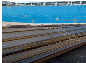
× H-beams bundled using single wire straps
